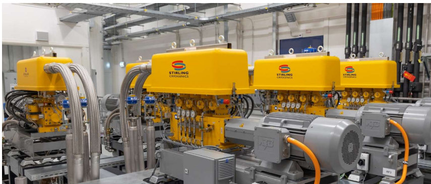
2019 Stirling Cryogenics Hydrogen Re-liquefier for Cold Neutron Source at RID Photo Courtesy Reactor Institute Delft, The Netherlands
